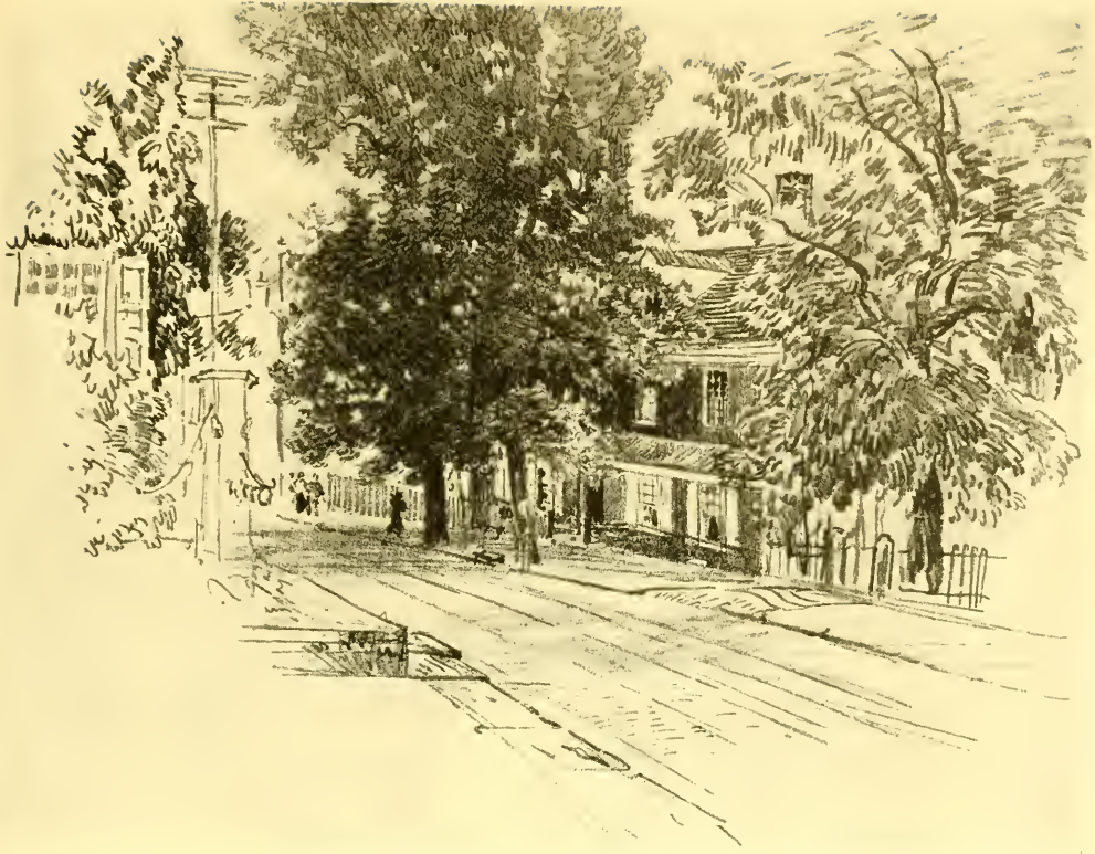
JOHNSON HOUSE, GERMANTOWN
